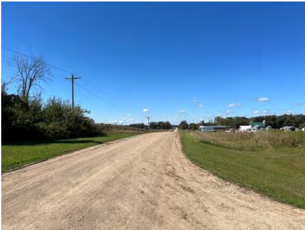
Looking west down 300 th St
