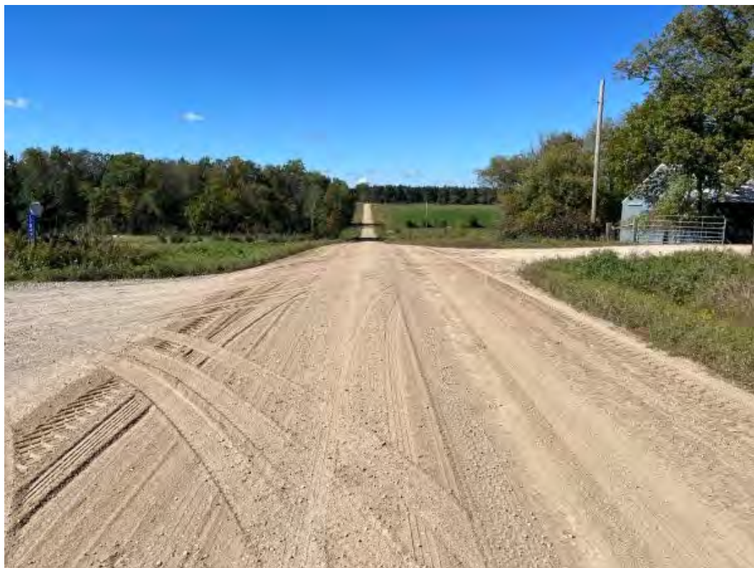
Looking west down 352 nd St
