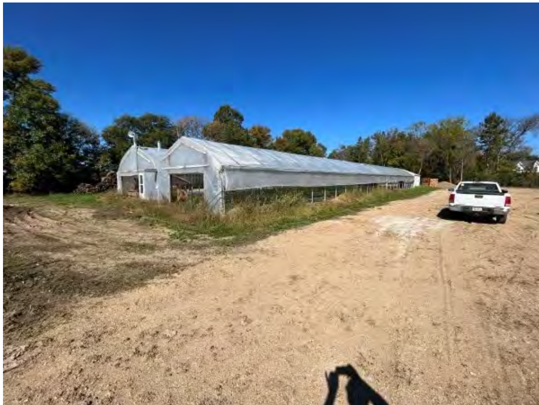
Existing greenhouse structures
